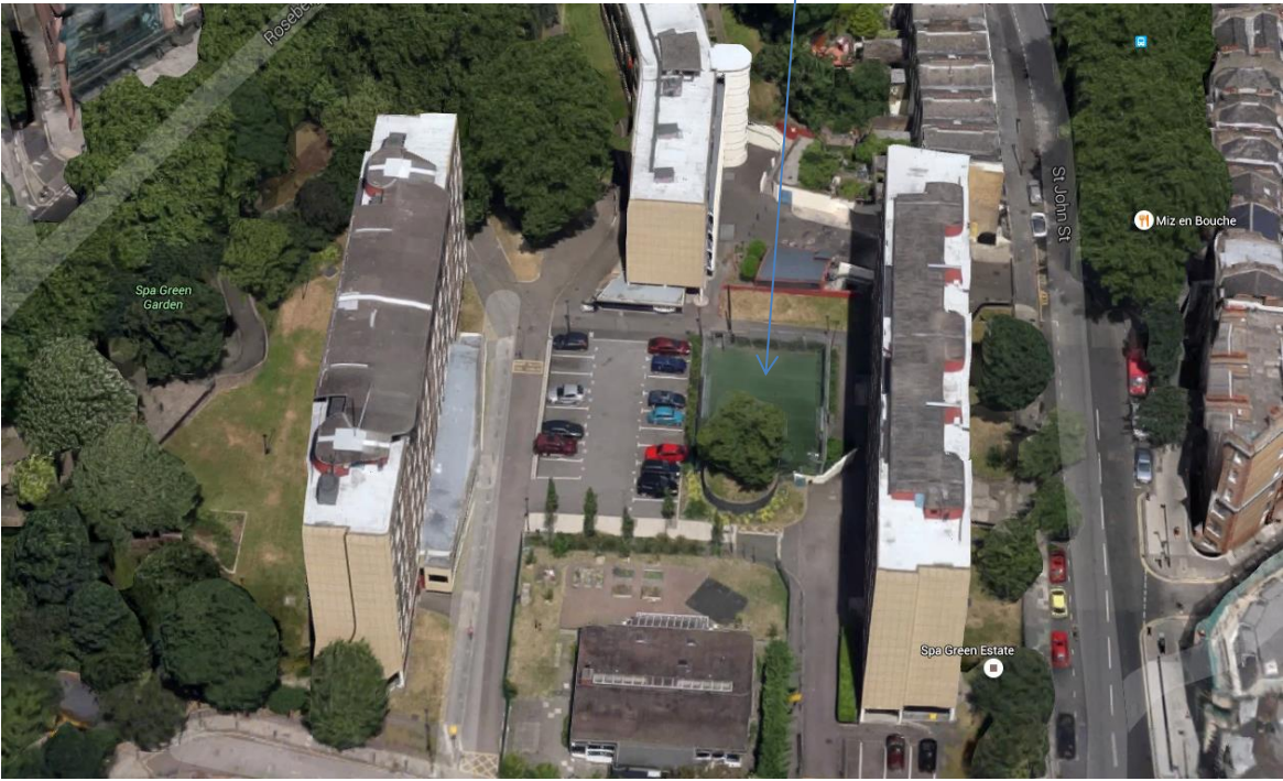
Image 1: Aerial view of the site
